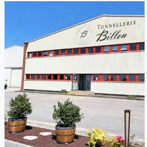
Renovated Billon cooperage facade.
