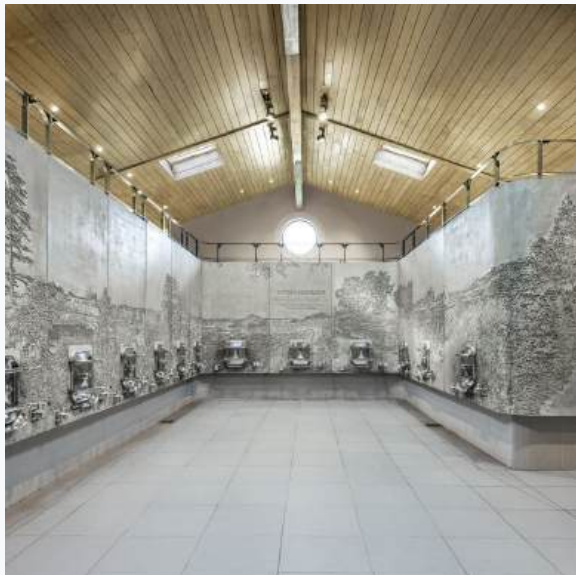
14 Tailor made Standard tanks custom embedded for Château Beauséjour Duffau Lagarrosse in Saint Etmillion.
