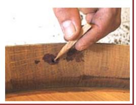
**4.** Then use a wood chisel to cut off the excess spile material. The blade of the chisel should be face up to make a clean cut. If necessary, smooth the exposed spile ends with sand paper to make a nice, clean finish. *Done!*
