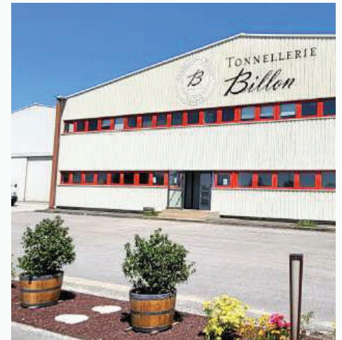
Renovated Billon cooperage facade.
