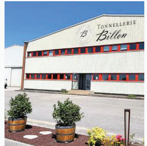
Renovated Billon cooperage facade.
