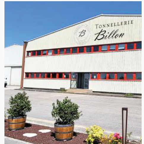
Renovated Billon cooperage facade.
